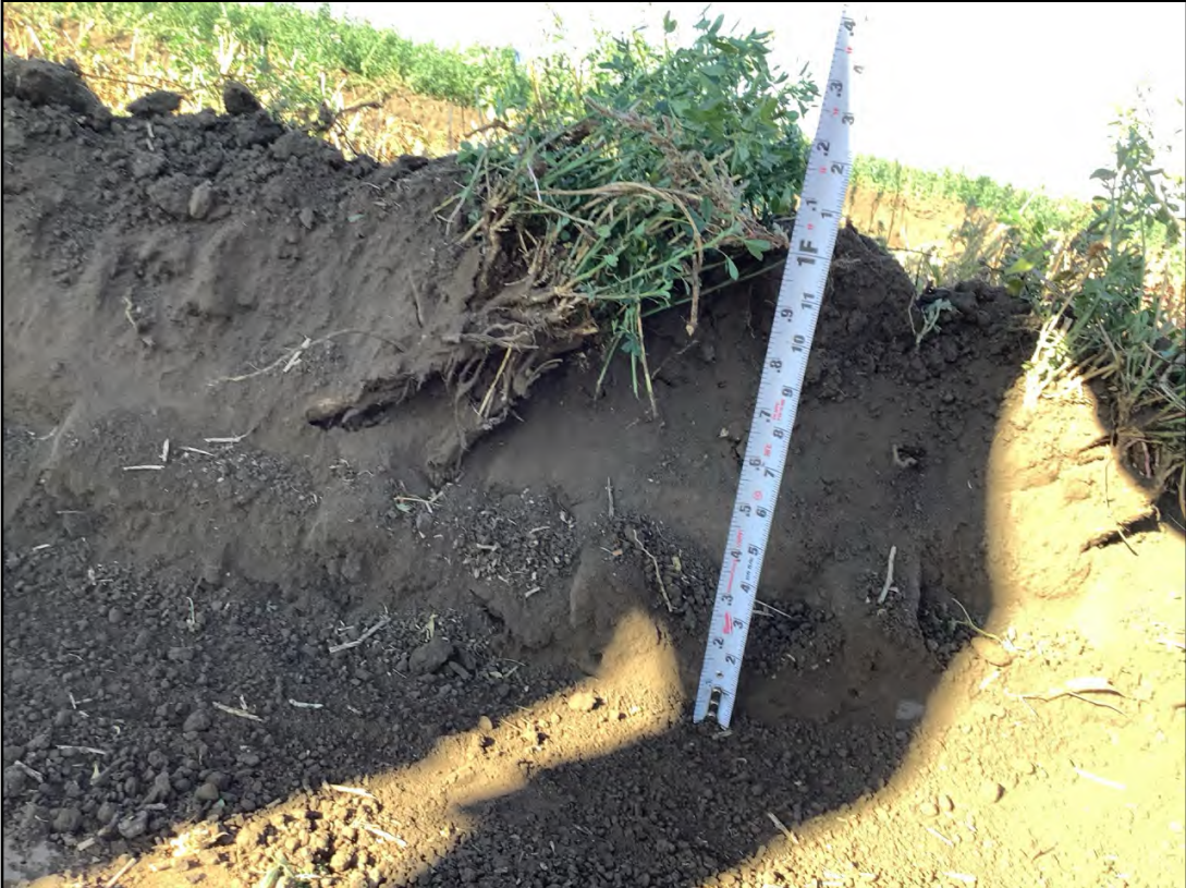
Point 10 Wind turbine site 1 Windrow of excavated topsoil placed on eastern border of site 1
