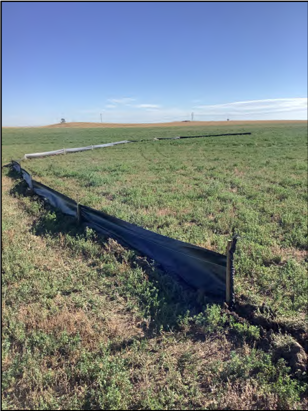
Silt fence installed on downslope of site.
